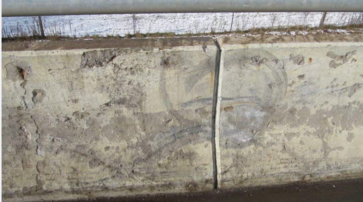
View of a wheel imprint in the wall of the overpass at the area of impact on Vanneck Road.
