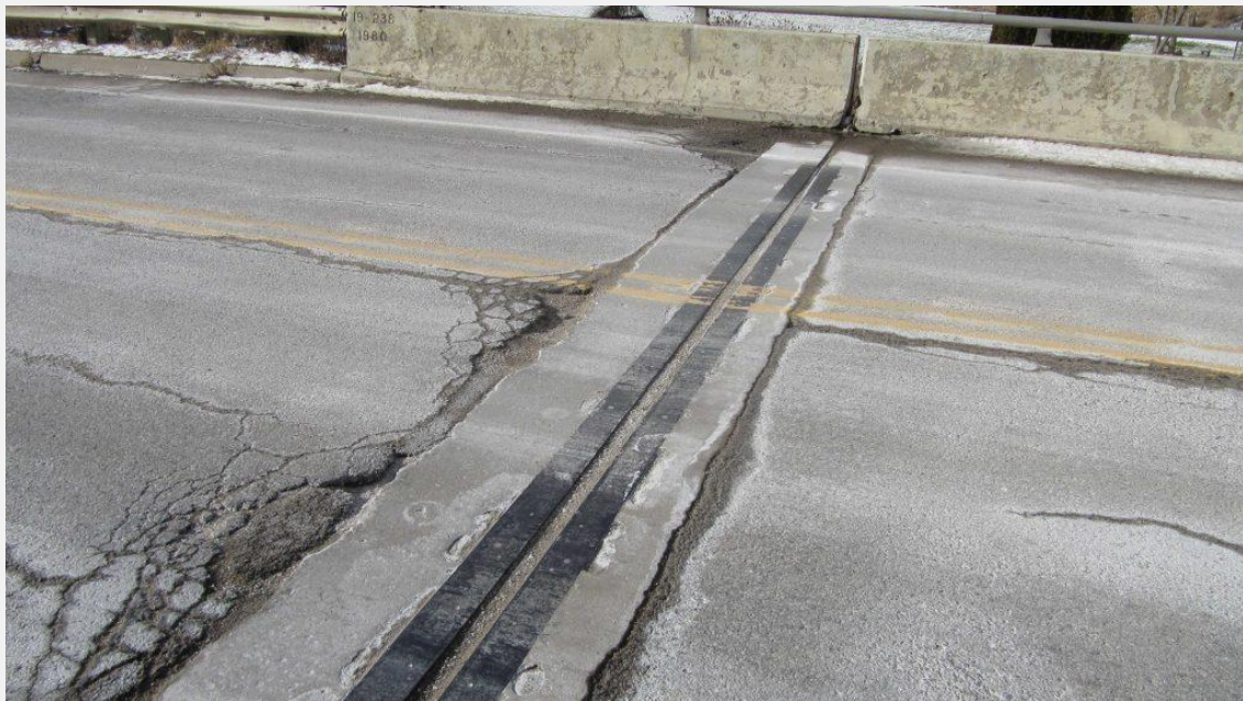
View of the aged condition of the south junction to the overpass where the loss-of-control took place. With a low tire force such disruptions of a vehicle's motion can contribute to a loss-of-control.
